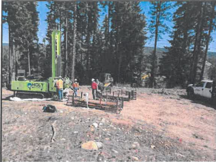
Drilling operations at borehole B-6 in Area 1
