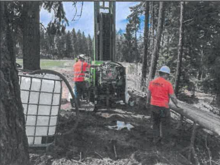
Drilling operations at borehole B-10 in Area 1
