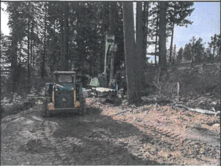
Drilling operations at borehole B-8 in Area 1
