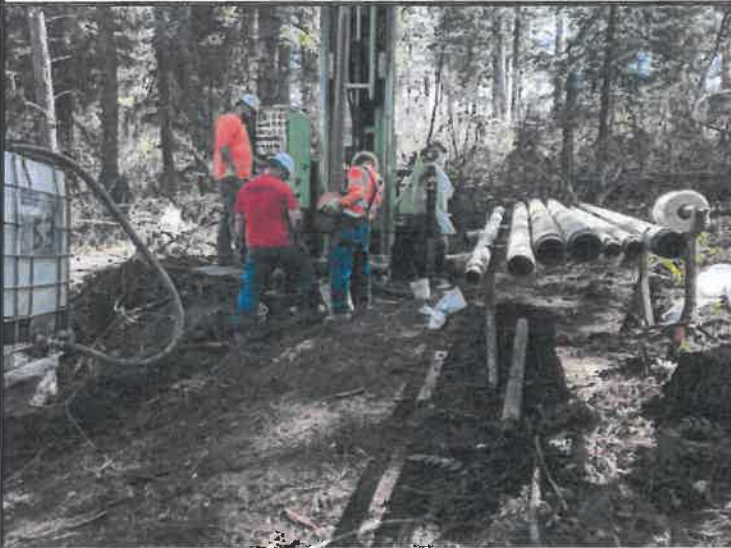
Drilling operations at borehole B-13 in Area 2
