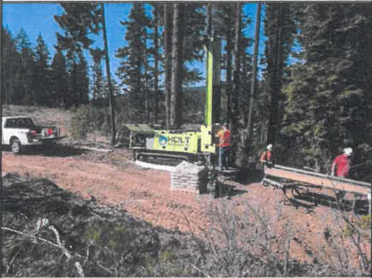
Drilling operations at borehole B-7 in Area 1
