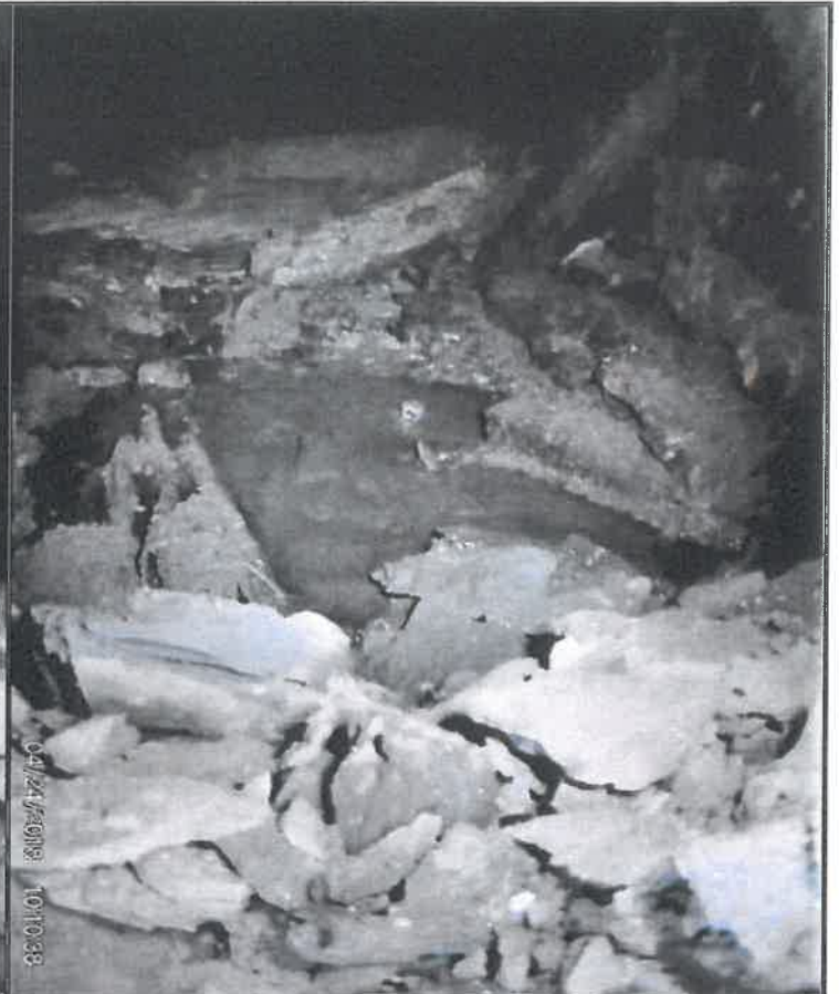
Floor of open mine shaft within boring B-8
