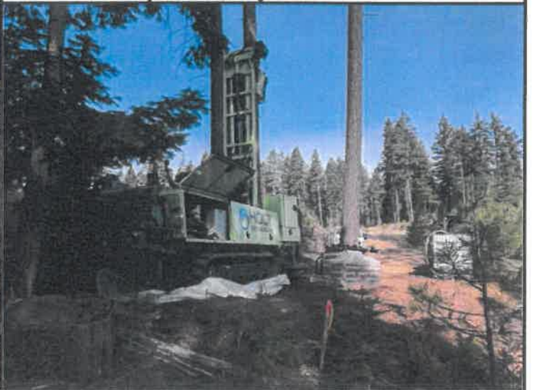
Drilling operations at borehole B-8 in Area 1
