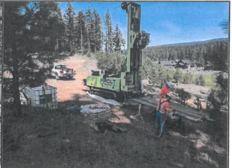
Drilling operations at borehole B-9 in Area 1
