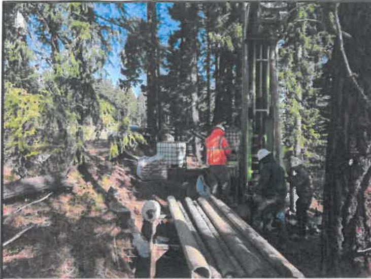
Drilling operations at borehole B-12 in Area 2
